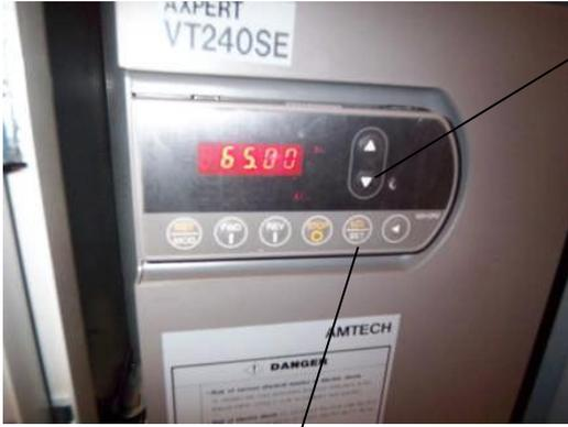
Push the Down Arrow Button to lower the Number, one digit at a time, down to zero. Note: You must change the speed slowly, one digit at a time or the drive will overload.
