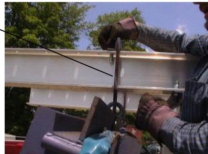
Make sure that the hoist support brackets are mounted as close to the front tires and vertical support beams as possible. Additional holes are provided in case the hoist has to be moved out further from the tank wall so the cables can clear vents or other obstructions. When the hoist is moved out, additional counter weights will have to be added to the back end of the fixture. Bolt the brackets down to the beam with (4) 5/8” “Grade 5” bolts.
