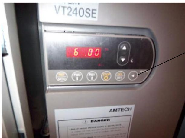
Push the Arrow Button to move the flashing digit to the digit to the right of the six.
