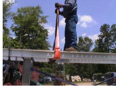
Use two straps to lift the fixture (one on each beam). Locate the straps about two feet back from the front vertical beams. Double wrap each strap so it won't slide along the beam during the lift. Pick the fixture off the ground, (if it tips either way, re-adjust the straps so the unit picks up level). Caution- make sure the crane and straps are sized properly for the load. The fixture and the hoist weighs around 2000 lbs.
